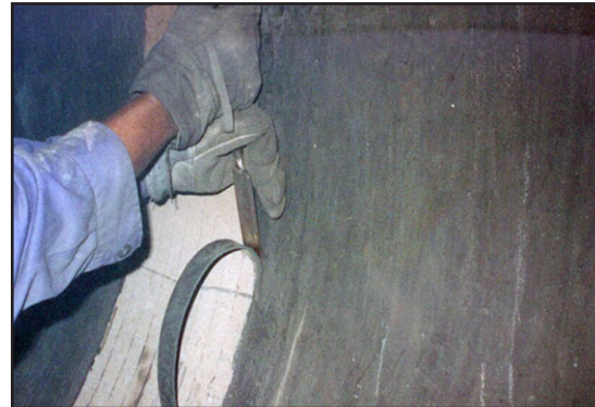
Rubber lining removal before cleaning
